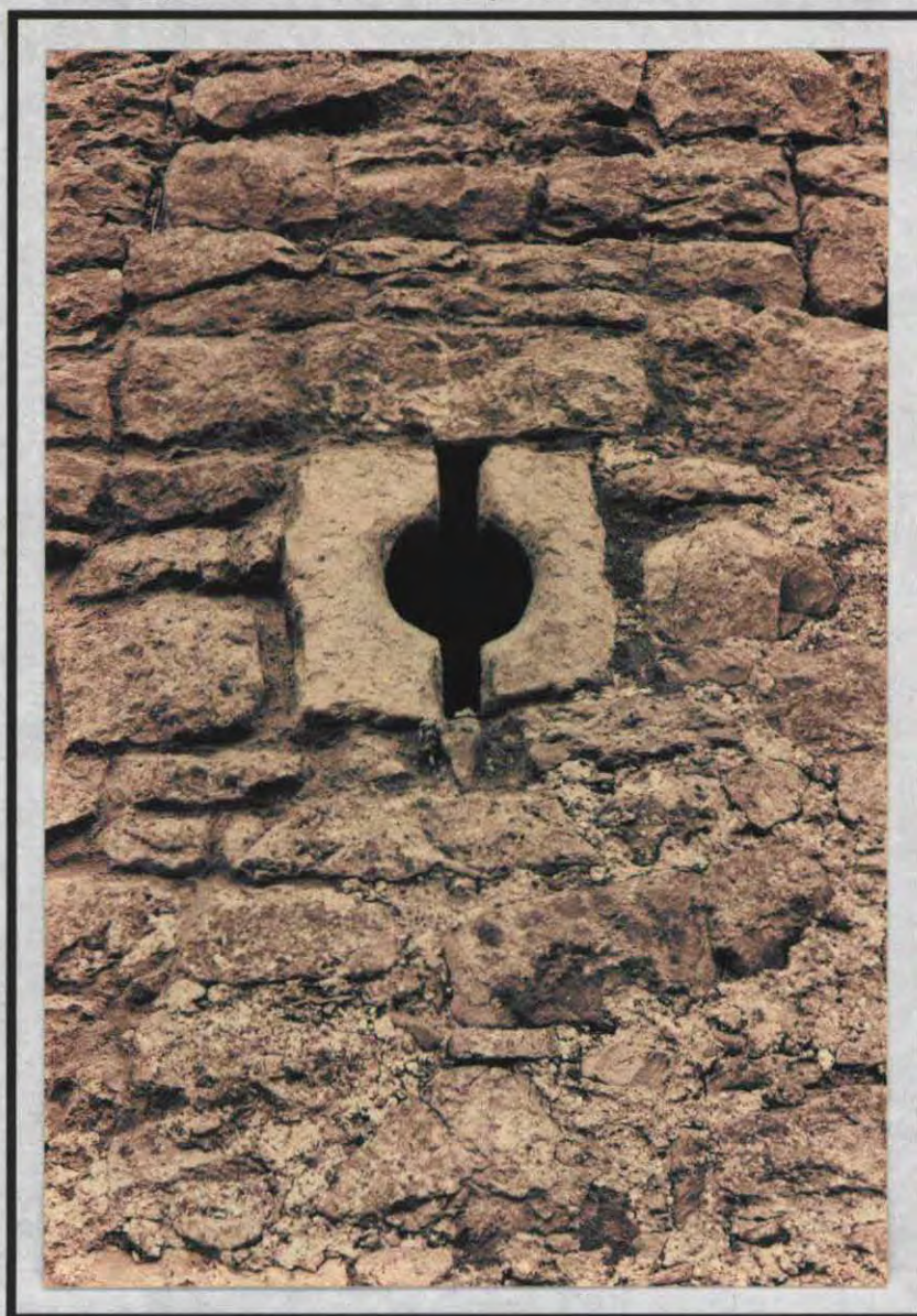
Plate 31: Detail of gun-port, tower house, Golden
