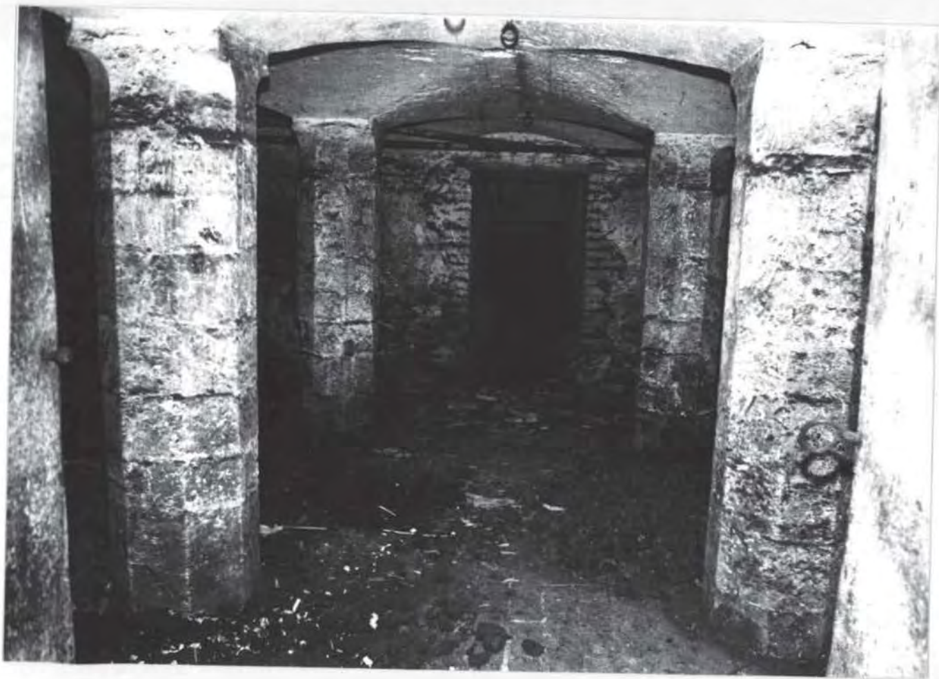
Fig. 33. Basement support pillars under the chapel (now the ballroom), probably 17th cent.
