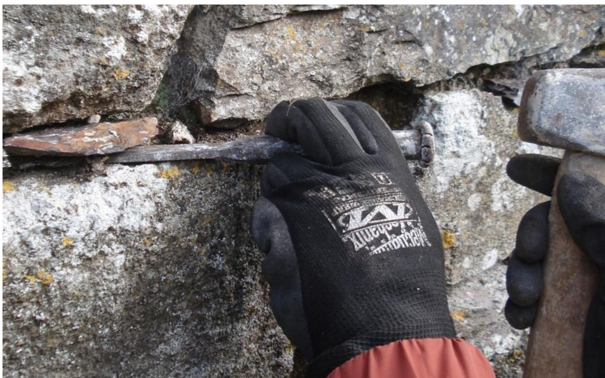
Plate 5: Raking out a horizontal joint using a plugging chisel.
