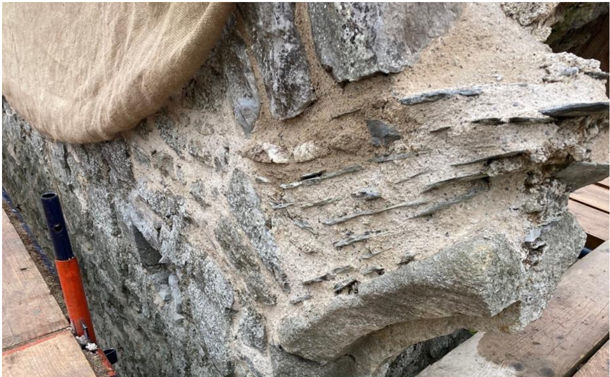
Plate 19: New mortar with slate pinnings, 'beaten back' and showing aggregate. Protective hessian in place, to drape over and protect the new work.
