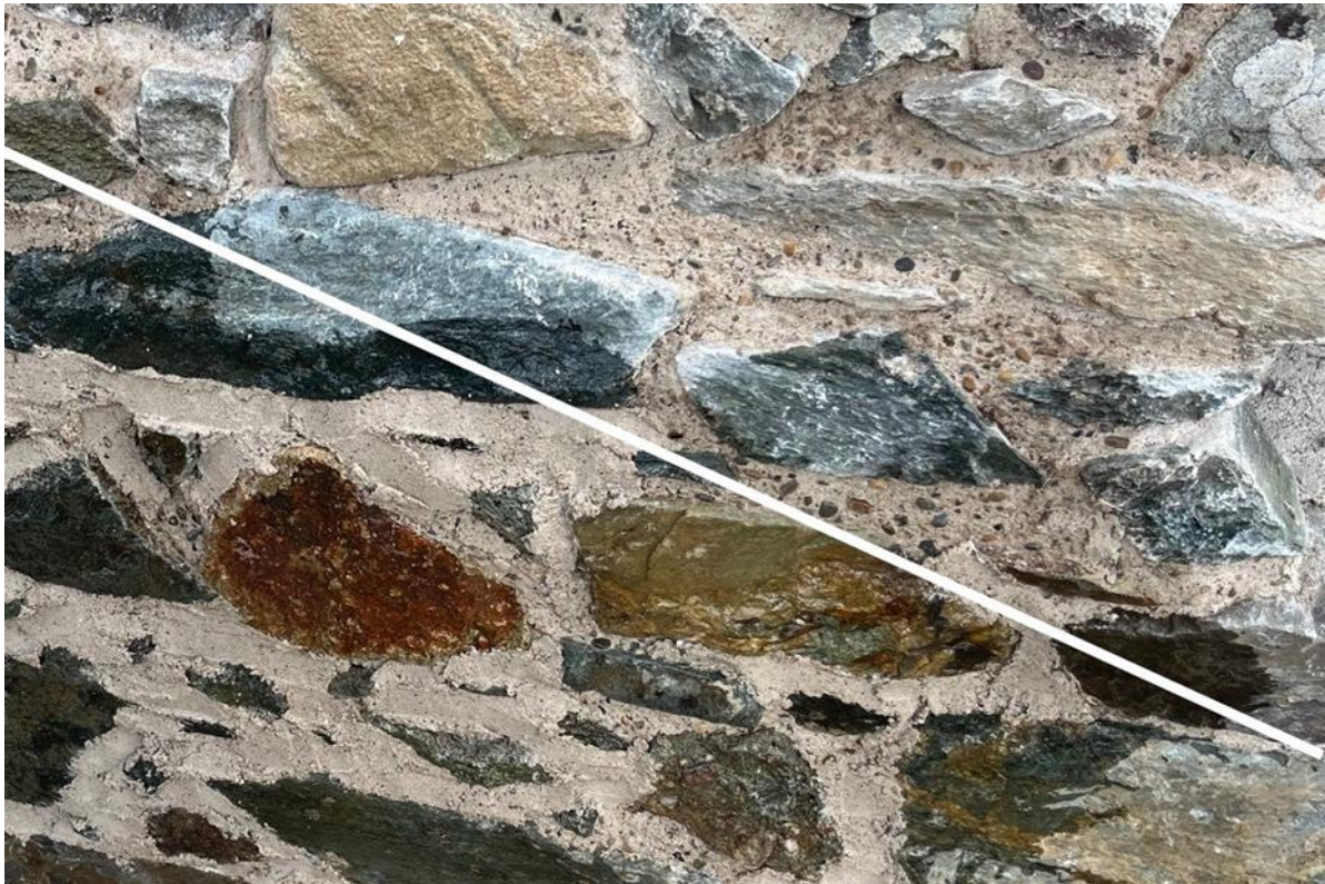
Plate 18: Fresh mortar below the white line. Mortar above the white line has been beaten back to expose aggregate, pinnings and the edges of the rubble stones.
