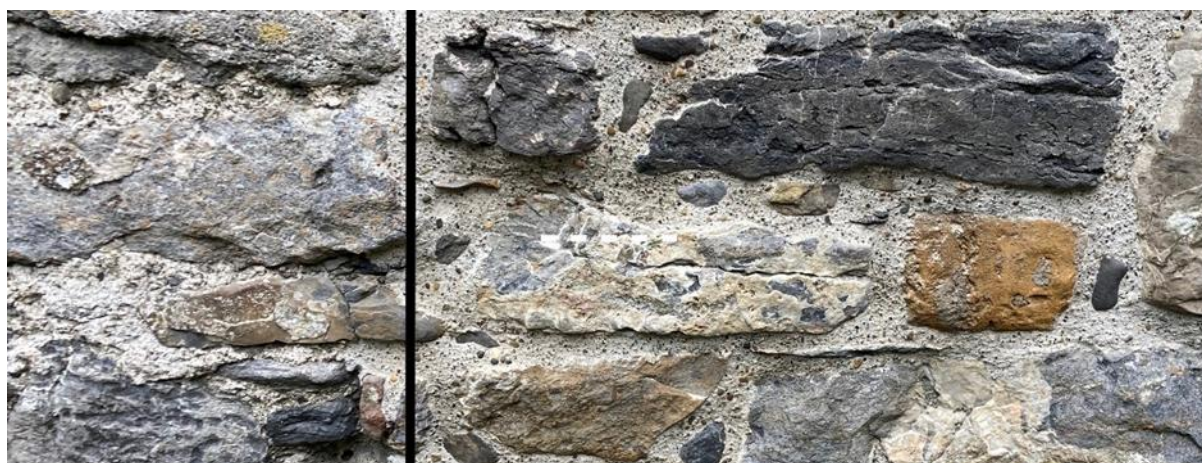
Plate 20: Agreed sample of new mortar and pointing. Surviving mortar to the left of the black line and approved new work to the right.
