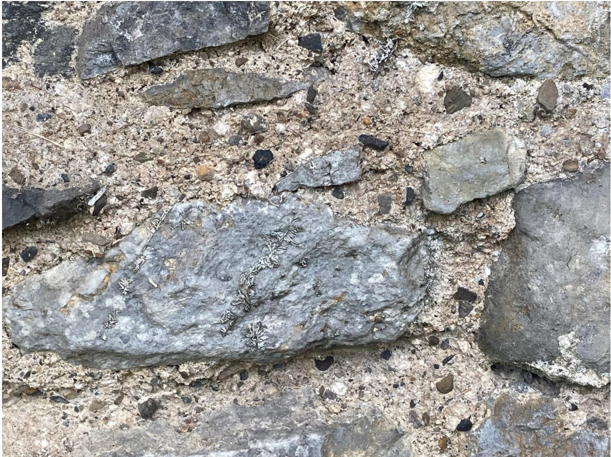
Plate 1: Surviving mortar, probably original, in good condition. Note the pinnings; large stones inserted to reduce the size of the bigger joints and to compress the mortar. Note the size and colour of the other stones, and how they affect the colour of the mortar.
