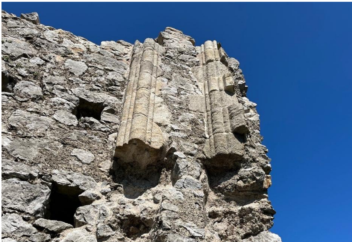
Plate 24: Window surrounds with fine joints and fine mortar, in comparison with the coarser mortar elsewhere on the structure.
