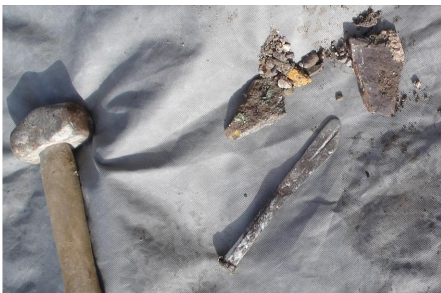
Plate 6: Pinnings and material raked out from the horizontal joint collected on the clean groundsheet.
