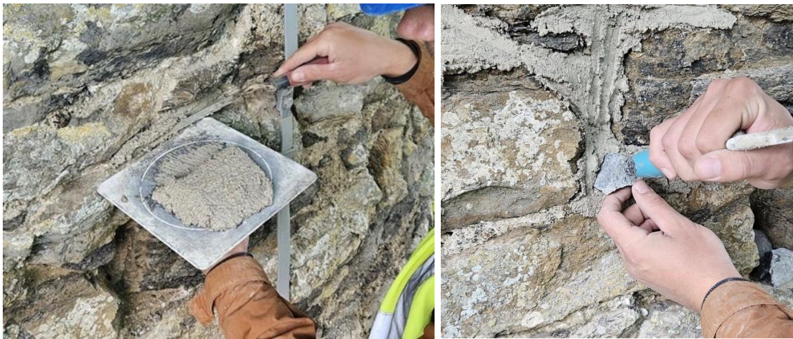
Plates 13–15: Dampening the joint, filling using a pointing iron and small hawk; inserting pinnings by tapping into place.
