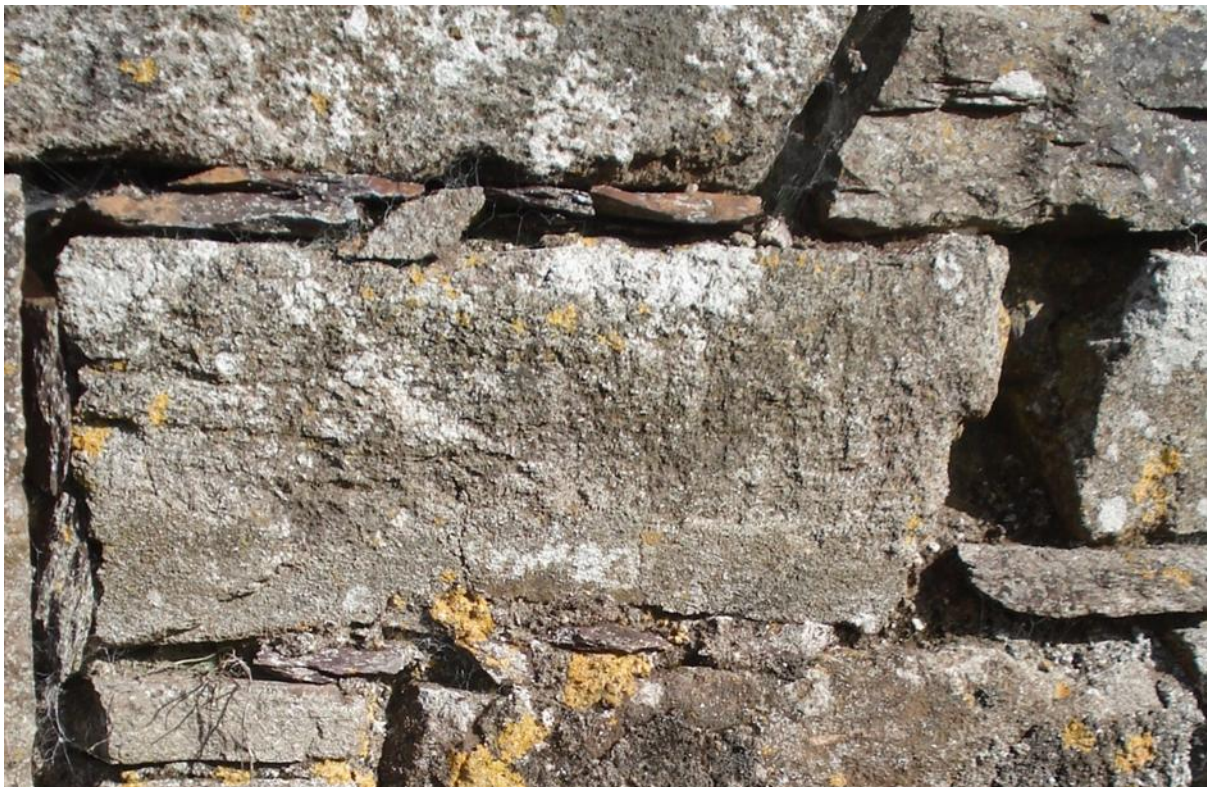
Plate 4: Joint ready for raking out of defective mortar.
